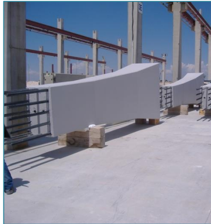
TAPUSA - FOOTBRIDGES OVER M-30 - MADRID – SPAIN STEEL TRUSS GIRDER OVER PRECAST CONCRETE PIERS SPAN LENGTH = 90 m
