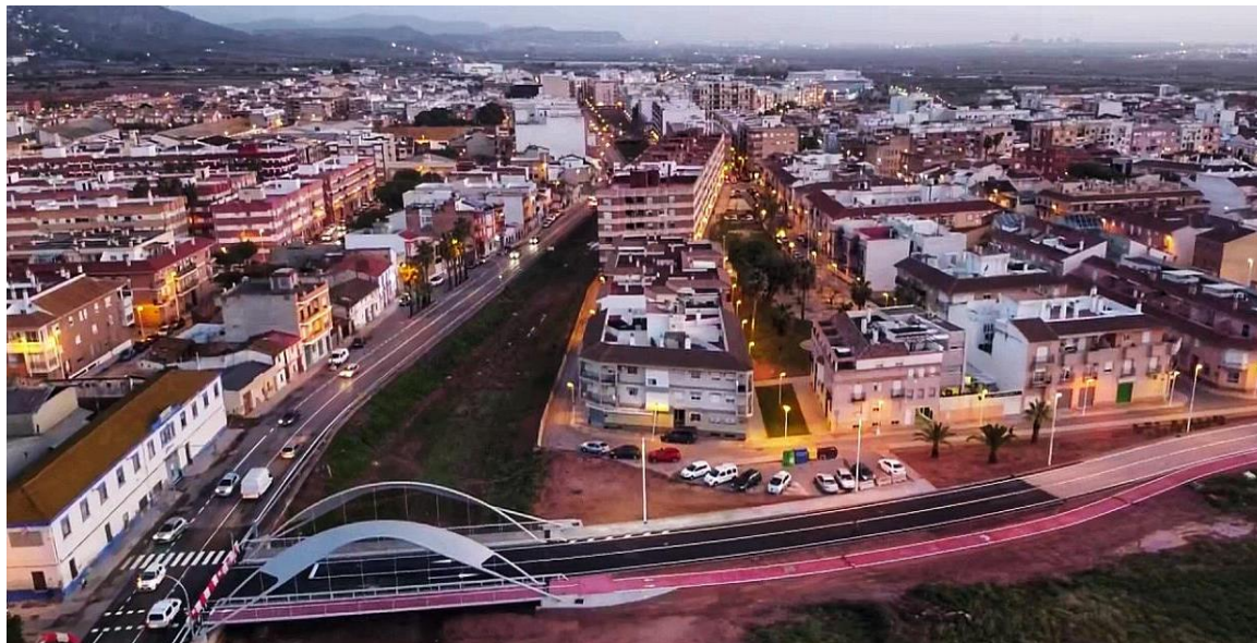
TAPUSA- ACCESS BRIDGE FROM CV-3307 TO THE RESIDENTIAL AREA OF "LA BARRACA" OVER THE "BARRANCO DEL VADO DE PUÇOL" – VALENCIA - SPAIN
